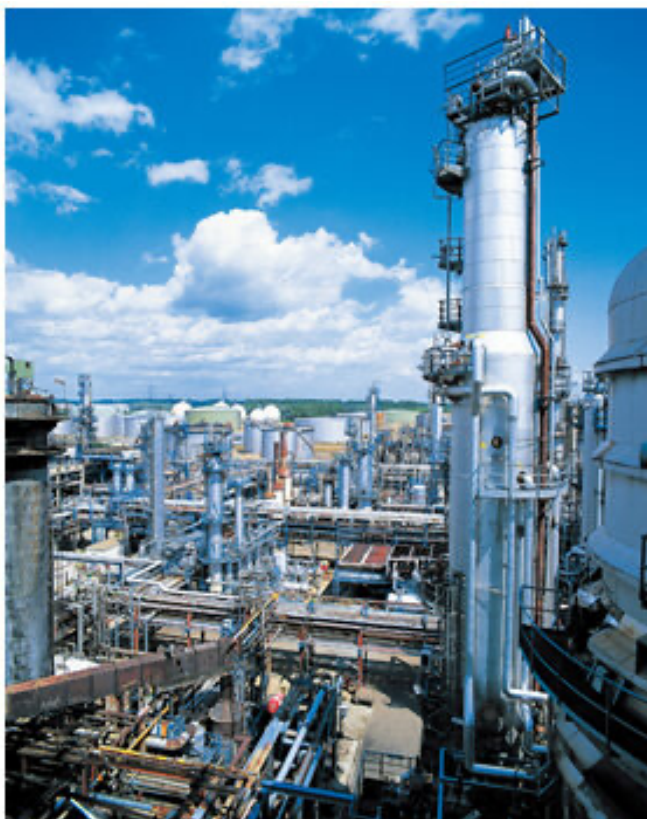
Hydro Carbon Processing Plant
